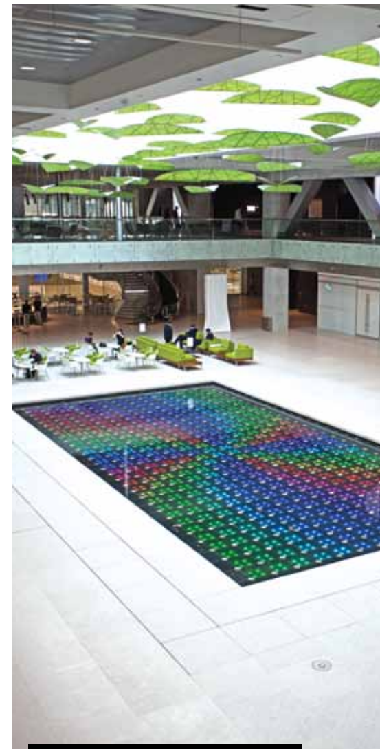
It is both the satisfaction of job well done, such as this light installation at the Qatar National Convention Centre, as well as the feeling they are contributing to the growth of their country in a meaningful way, that inspires Techno Q’s directors Al Jaidah and Al Ansari to action. (Photo courtesy Techno Q)
